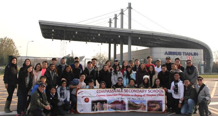
Tianjin Airbus Final Assembly Line
